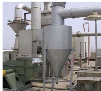
Fig 7: Cyclone Separator
