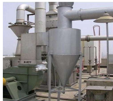
Fig 7: Cyclone Separator
